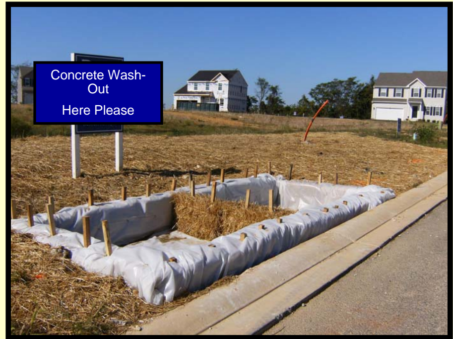
Concrete Wash-Out
